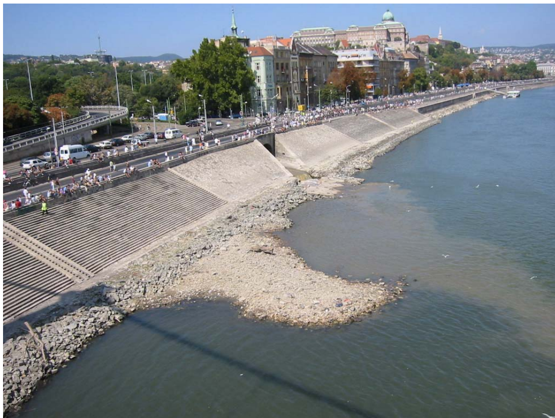
Figure 1: The mouth of Ördögárok ('Devil's ditch') at the Elizabeth bridge. Both the arriving sewage and the dam dike that turns the untreated sewage towards the main current are well visible because of the low level of the water.
