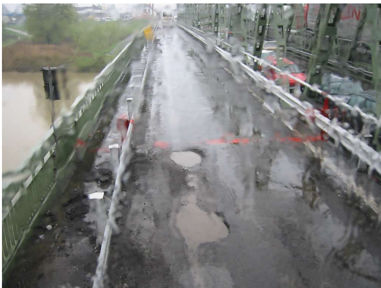
Figure 2. Pavement quality discontinuity. One can physically distinguish the two sides of the future Schengen border at the middle of the bridge over the river Tisza between Záhony and Chop. (Sorry for the quality of my rainy photo)
